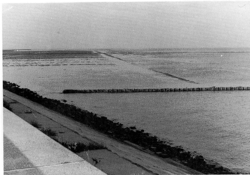
Fig. 1.8. Marsh restoration works, Deal Hall, Dengie Peninsula, Essex.
