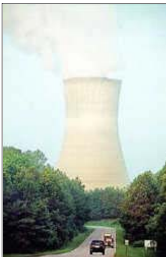
A tower rises at the Shearon Harris nuclear plant, 25 miles from Raleigh.
