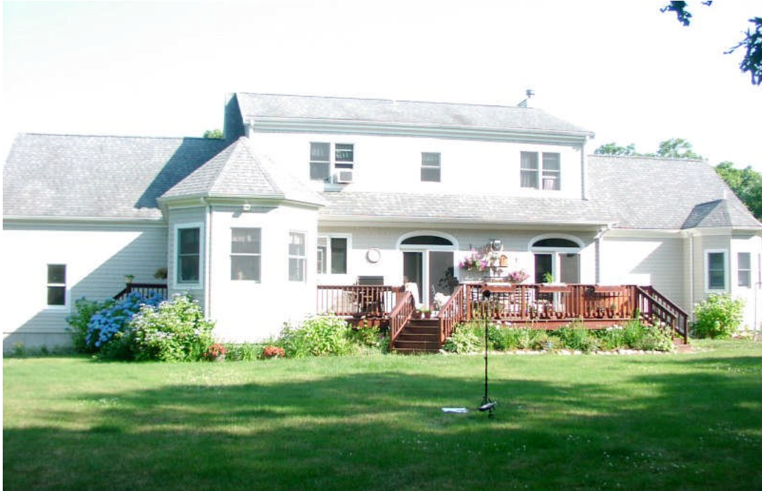
Figure 25 Photo of Site ST-4 Position 2, 30 Durham Rd
