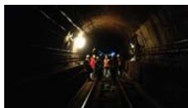
Subway Tunnel to Close
