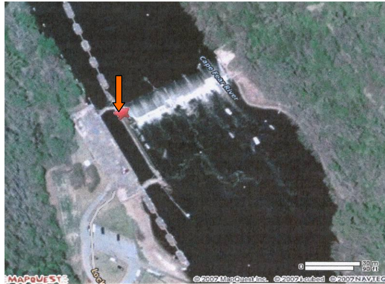
Figure 2. Aerial photograph of Lock & Dam #1
